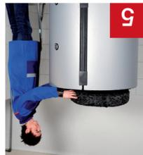
Insert the ECO SKIN rondelles at the top on the boiler and position by pressing down slightly.
