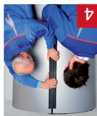
After attaching the cover installation strip, the ECO SKIN insulation can be sealed using the second hook closure strip.
