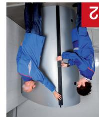
Afterwards, pull the perforated insulated part with the geomembrane inward over the connections.
